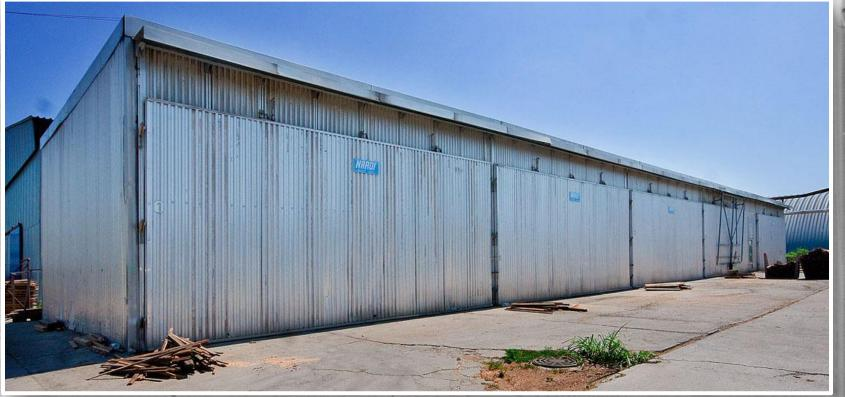
Type -convection drying 740 m3 one-time loading volume ( 8 chambers )
