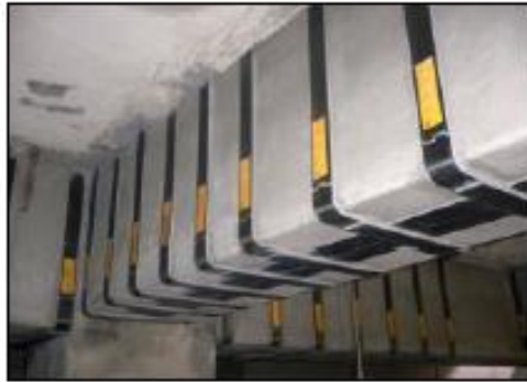
Carbon laminate system of external reinforcement
