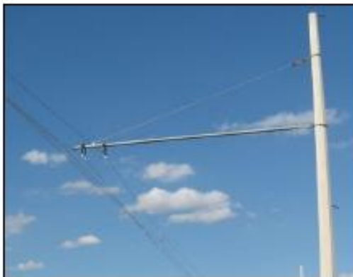
Bracket overhead catenary for trolley
