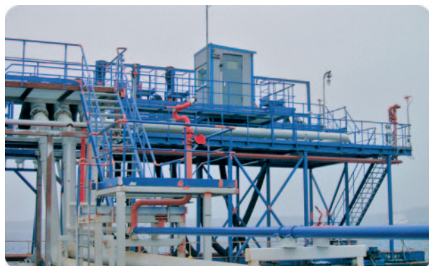
The berth complex for reloading of the oil products of the Vitino-sea berth on the White Sea
