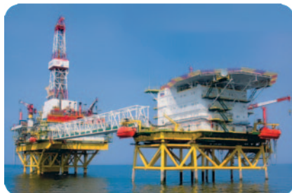
Oil platforms "Kravzovskoye", Kaliningrad region
