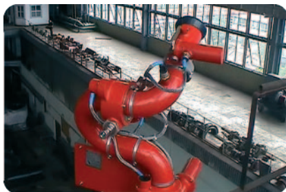
Fire robots in Petrozavodsk HPP machinery hall
