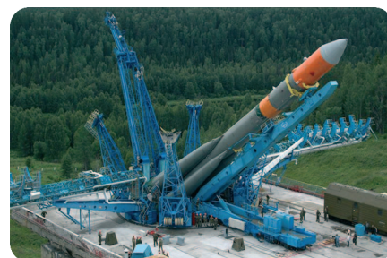
“Plesezka”-launch-vehicle site, test facility
