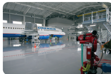
FR Fire robots protecting an airplane hangar, Russia, Orenburg city
