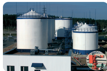
Reservoirs and r.r.-viaduct “TNK”, Petrozavodsk-city
